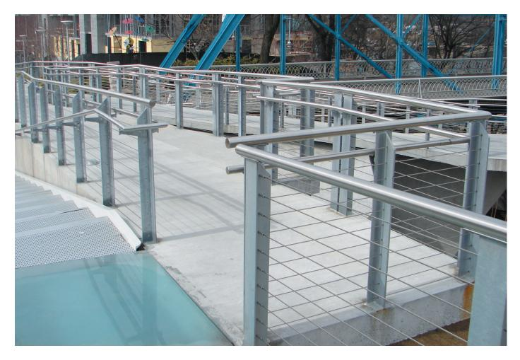
lines, each tensioned to a minimum of 225 lbs. over a height of 36" to 42". The posts to which hardware is mounted must be constructed so that they will not deflect perceptively as the cables are tensioned to loads of 225 lbs. or more. All of these variables work together to minimize the deflection of the cable so as to not allow a 4" sphere to pass between the cables when they are properly tensioned in a welldesigned frame.
