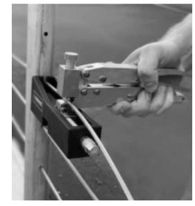
**4.** Connect the cable at the end post, without having to pull tension through the entire cable length, only from the pre-tensioner to the end post. After installing the cable at the end post, release the clamp and remove the pre-tensioner. Reset using the impact driver, and move on to the next cable, repeating the process.
