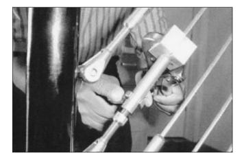
**6.** If tensioners are mounted to tabs, structural tees or lag eyes, tighten the mounting screws.
