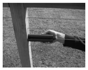
**2.** Clamp the correctly-sized locking pliers to the cable, so the shaft beyond the thread fits into the counter-bore in the locking pliers.
