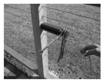
**5.** You may now connect your cable at the last post (end post), without having to pull tension through the entire cable length, just from the pre-tensioner to the end post. When you have finished installing the cable at the end post, release the locking pliers, remove the pre-tensioner, and move on to your next cable, repeating the process.
