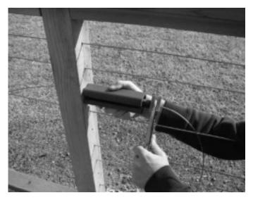
**4.** Using a 3/4" wrench on the wrench flat of the all-thread, rotate the all-thread counter-clockwise, tightening the cable to the desired level of tension.
