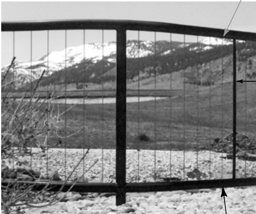
DRILLED HOLES TO ACCEPT INVISIWARE® RECEIVERS
